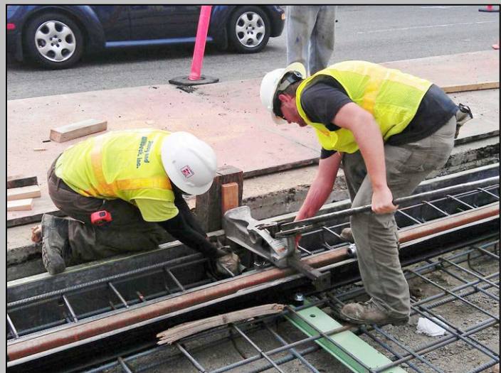
Using a track jack to align the rail
