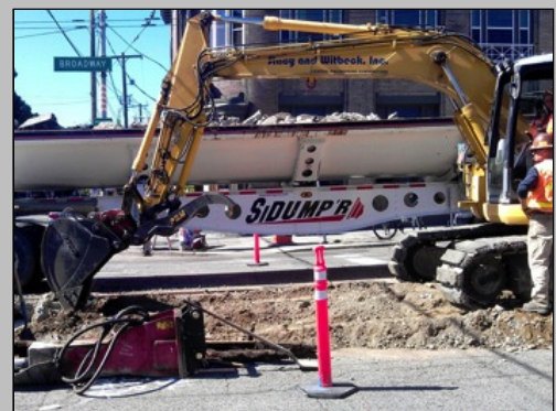
Excavation on Broadway at Pike
