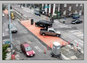
Steel plates cover excavated trackway at Broadway and Union. Concrete is poured on weekends during low traffic periods.
