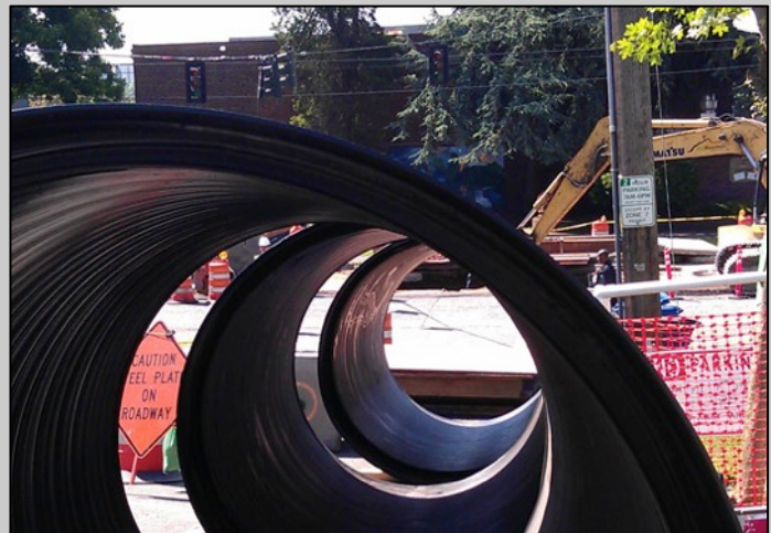
72" Storm Drain Pipe Ready for installation at Broadway and Yesler
