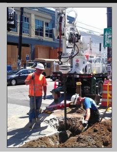
Constructing Pole Foundations To install new signal poles a 3' diameter hole is augured 12' deep then reinforced with steel and filled with concrete.
