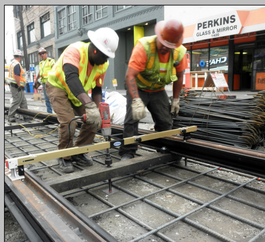
Adjusting rail to final grade
