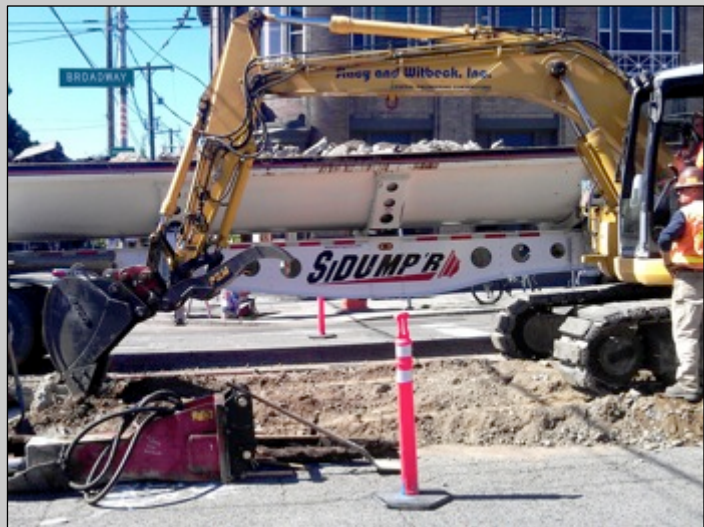
Excavation on Broadway at Pike
