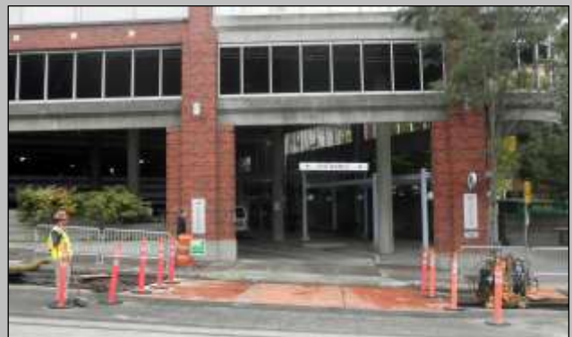
The project maintains access to businesses during construction. Here is an example of this at The Polyclinic on Broadway.
