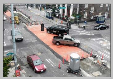
Steel plates cover excavated trackway at Broadway and Union. Concrete is poured on weekends during low traffic periods.
