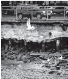
Seawall failure (courtesy Seattle PI archives, 1986)
