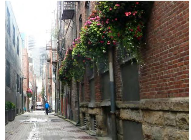
Each paver should be dimensioned exactly the same with tolerances of no greater than 3/32". As is currently the case in the historic alley paving, pavers should be set on their narrow edge (approximately 2" by 8") so that a narrow running bond pattern is visible on the finished alley surface. This reproduces the historic pattern of brick pavers within the alleys.
